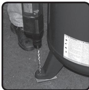
**Insert** mounting bolts. Use 3/8 inch x 5 inch wedge anchors to secure the unit. Place nut and washer on bolt. **Thread** nut onto bolt until tops are flush. **Strike** bolt with hammer until nut and washer are setting on top of the compressor foot.
