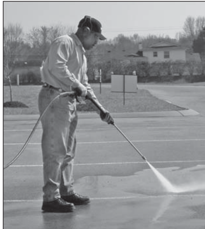
Figure 16 - Optimum angle to cleaning surface
