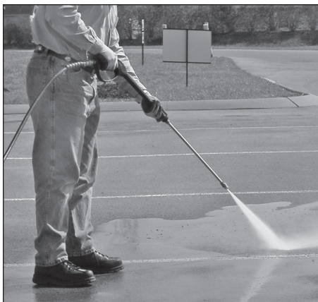
Figure 11 - Optimum angle to cleaning surface
