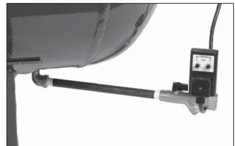
Figure 11 - Automatic Tank Drain
