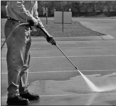
Figure 12 - Optimum angle to cleaning surface
