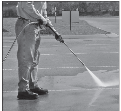
Figure 22 - Optimum angle to cleaning surface
