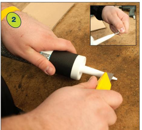
Prepare caulk tube. Read directions on the tube before cutting the tip and breaking the seal. Cut tip with razor knife at 45 degree angle. **NOTE:** For narrow bead, cut at tip. For wider bead, cut further back from the tip. Use a long nail to break the seal.
