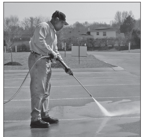
Figure 21 - Optimum angle to cleaning surface
