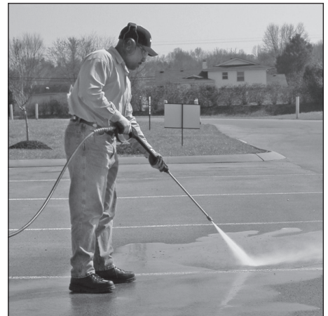
Figure 15 - Optimum angle to cleaning surface
